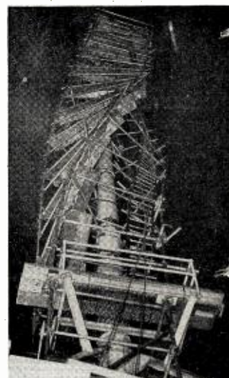
TWISTED WRECK is all that remains of the CBS New York FM antenna after the hurricane hit it. Antenna is 85 feet high and is located at 500 Fifth Ave., New York.
